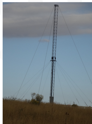
One of WWV’s Single Band, Half-Wave, Vertically Polarized, Center Fed Dipoles (aka: modified sleeve antenna).
