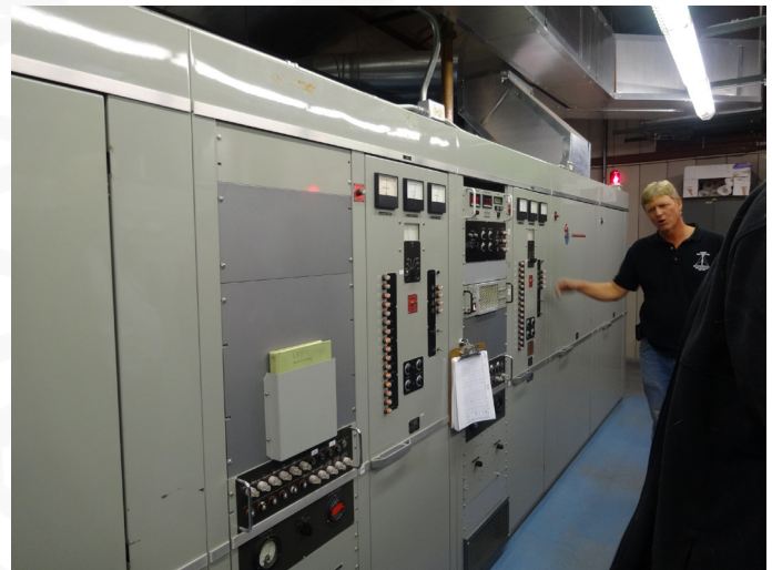
WWBV has three Continental Electronics 50 kW transmitters, two active and one standby.
